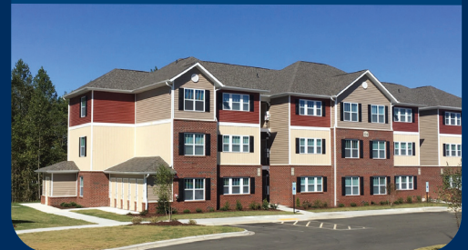
Mocksville Pointe Apartments, Mocksville, NC FGM Development | Mills Construction
